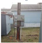
Most mobile homes have meters placed between properties on meter boards. The electric service lines from the meter to the home do not belong to the utility. They are "owner's wire" and will not be located by the utilities. Private locator contractor members of Miss Utility are listed on our website (www.missutilitydelmarva.com) under ABOUT US/MEMBER LIST/PRIVATE LOCATOR CONTRACTOR MEMBERS.
